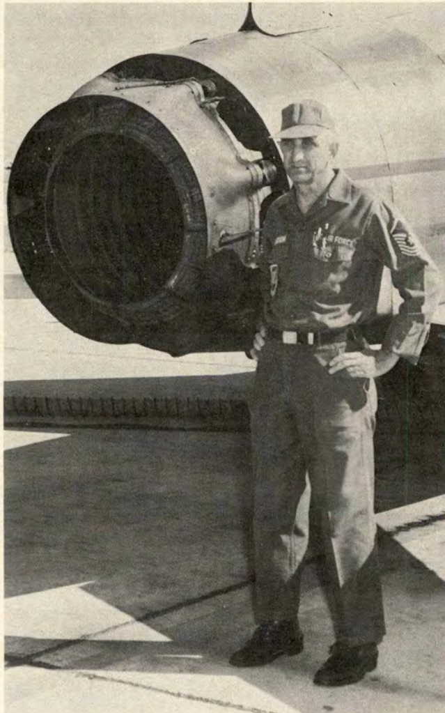
SMSgt Mike Suzich, Jr., stands beside a successfully transplanted -23 afterburner in one of his unit's F-100s.
